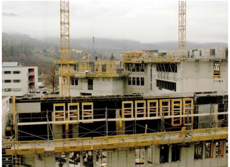
The IZW during the building phase in the Fall of 2006
