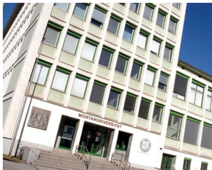
The RWZ as seen from the Erzherzog-Johann-Straße.
