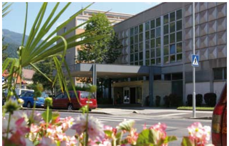
The old facade
