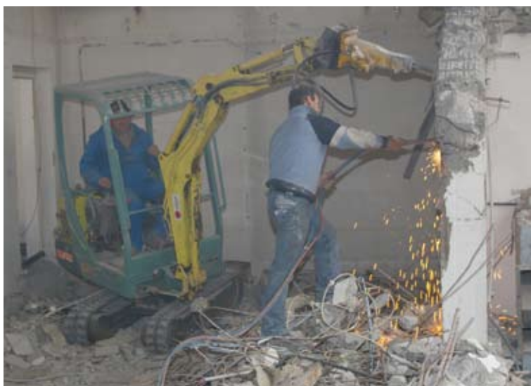
Heavy equipment gets to work on the old building fabric.
