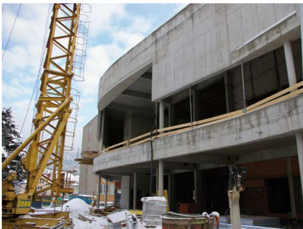
Work goes on even under winter conditions.
