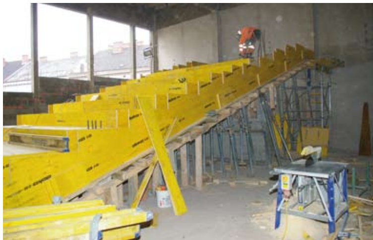
The new lecture hall takes shape.
