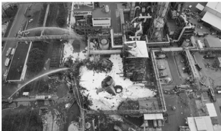
Fig. 1: Thermal runaway in tank # 3 at Currenta (Germany) in July 2021
