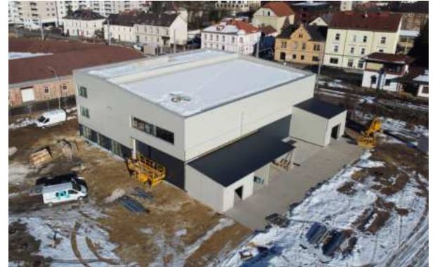
Figure 1: Hydrogen Research Centre
